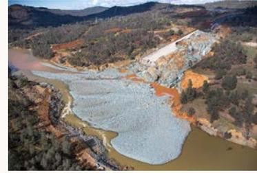
*Oroville Dam spillway incident occurred in 2017 primarily due to inadequate design for foundation conditions of the primary and emergency spillways. Incident resulted in evacuation of 188,000 people and yet to be quantified environmental and economic impacts.*
