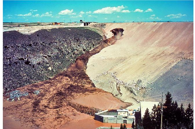
Figure 5. Image of Teton Dam failure [10]
