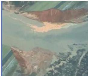
*Failure of Big Bay Dam in 2004 resulted in destroying 48 homes, washing out a bridge, and damaging 53 homes, 2 churches, three businesses and a fire station due primarily to inadequate seepage controls and recognizing warning signs.*
