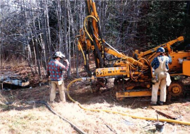
**Figure 5. Abandonment of a conduit by cement grout through holes drilled from the surface of the embankment dam to depths of up to 60 feet. [1]**
