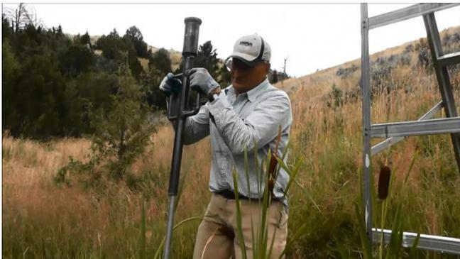
Photo 4: Installing Piezometer by Hand Auger
