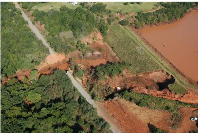
Figure 6 – Sugar Creek L-44 Spillway and Dam Erosion
