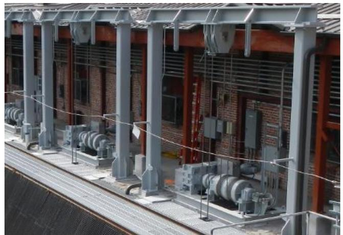
Photo 1: Wire Rope Hoisting Systems for Fixed Wheel Gates
