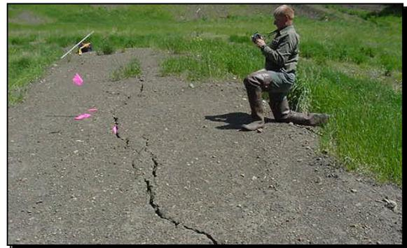
Photo 12: Longitudinal crest crack (Montana DNRC)
