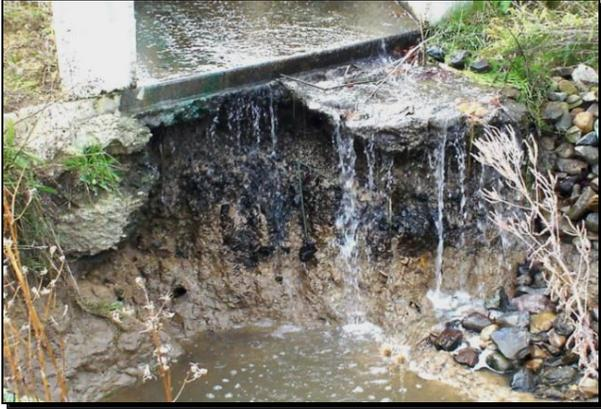
Photo 22: Erosion and undermining of outlet structure (AECOM)
