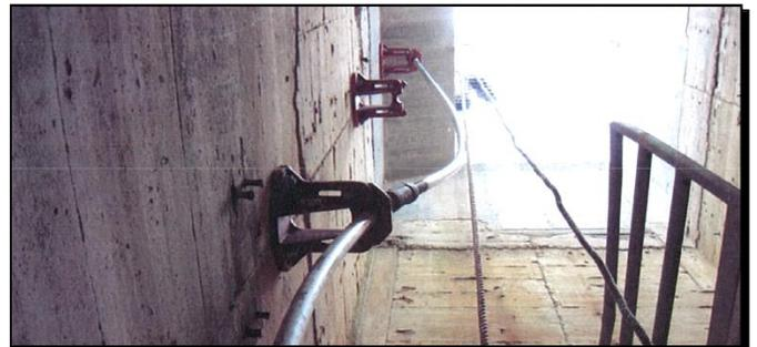
Photo 21: Bent gate stem (AECOM)
