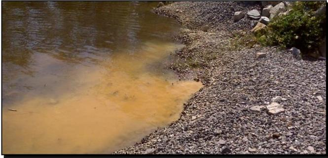
Photo 18: Muddy seepage at downstream toe (ASDSO)
