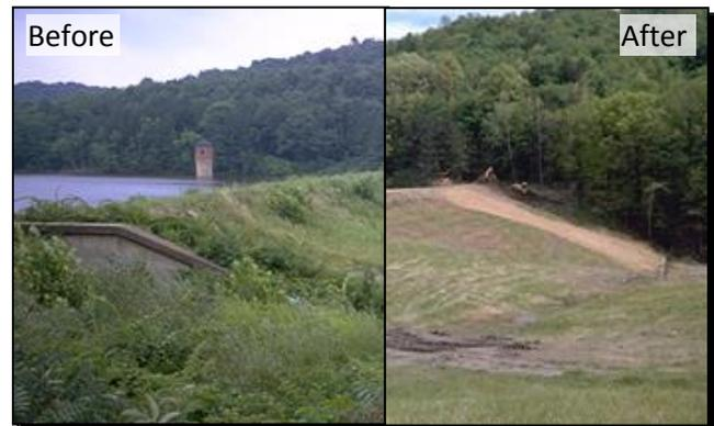
Photo 3: The importance of mowing before an inspection.
