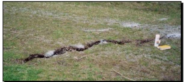
Photo 11: Transverse crest crack (ASDSO)
