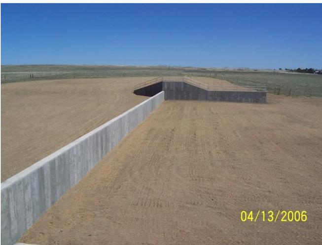
Figure 5: Sharp Crested Weir
