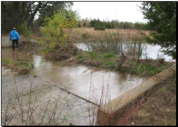
Photo 19: Vegetation obstructing spillway flow (AECOM)
