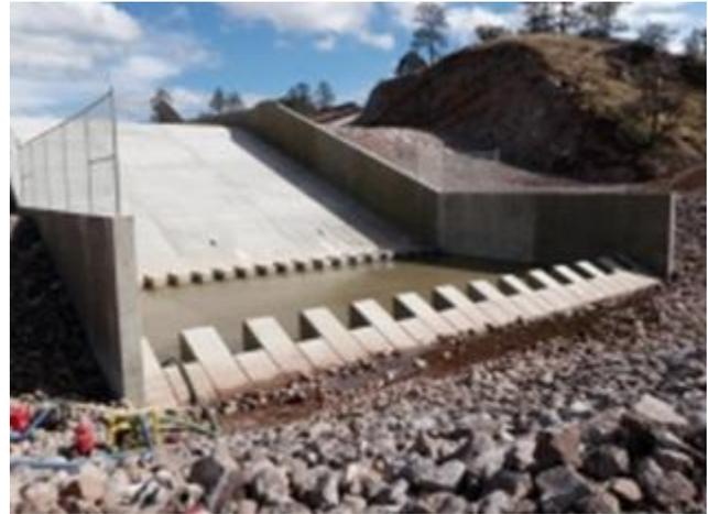
Figure 11: Lined Spillway Chute (Concrete)
