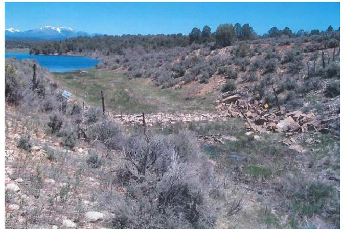
Figure 13: Unlined Spillway Chute
