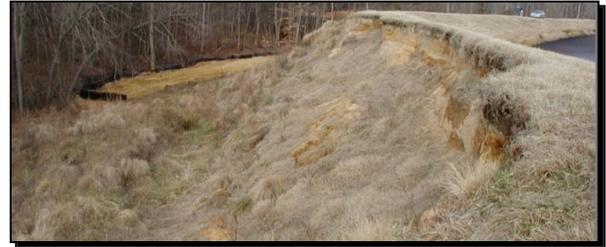
Photo 6: Deep slide, slump, and slips on a slope (ASDSO)
