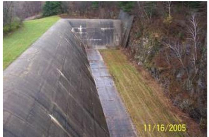
Figure 9: Side Channel Spillway
