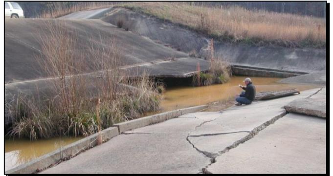
Photo 2: Failed concrete spillway following operation during a storm event.
