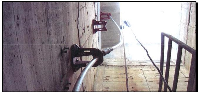
Photo 21: Bent gate stem (AECOM)
