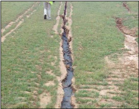
Photo 9: Slope erosion and sparse vegetation (AECOM)
