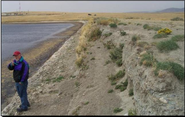
Photo 8: Loss of riprap and slope erosion (Montana DNRC)
