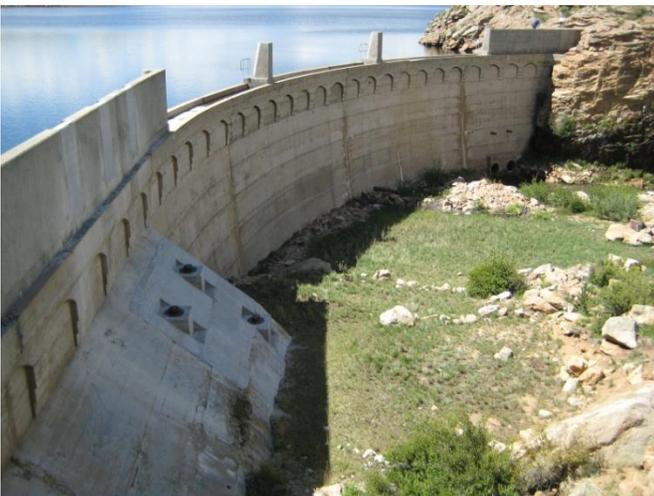
Figure 17 – Downstream Face of Tarryall Dam from the Right Abutment
