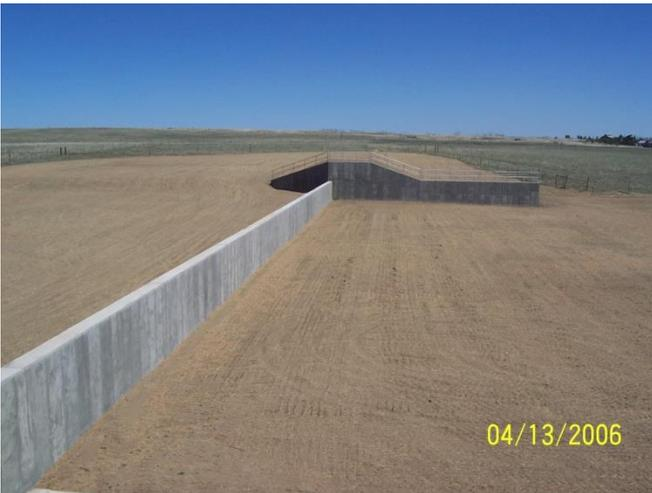
Figure 5: Sharp Crested Weir
