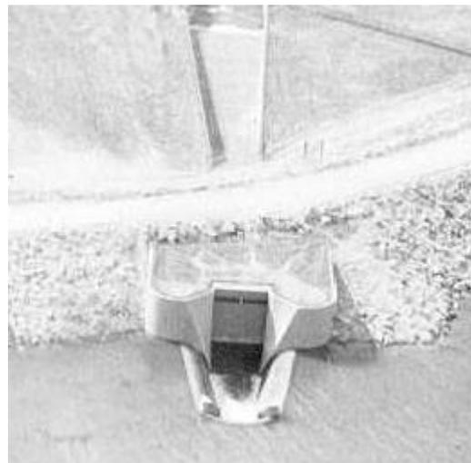
Figure 10: Bathtub Crest Structure (Reclamation 1987)
