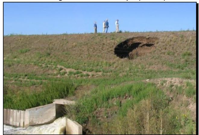
Photo 7: Sinkhole on downstream slope (AECOM)
