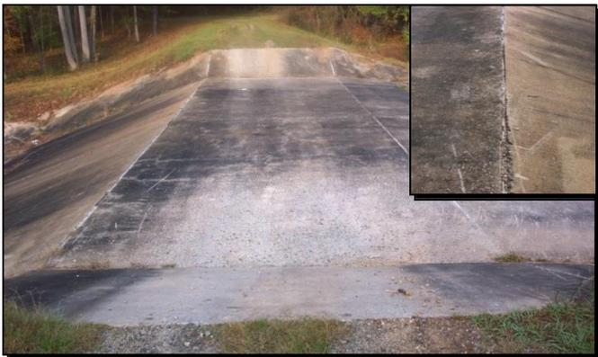
Photo 1: Concrete spillway from the inspection report. Photo inset shows an open joint.
