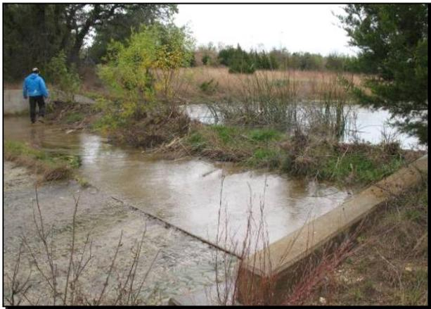
Photo 19: Vegetation obstructing spillway flow (AECOM)
