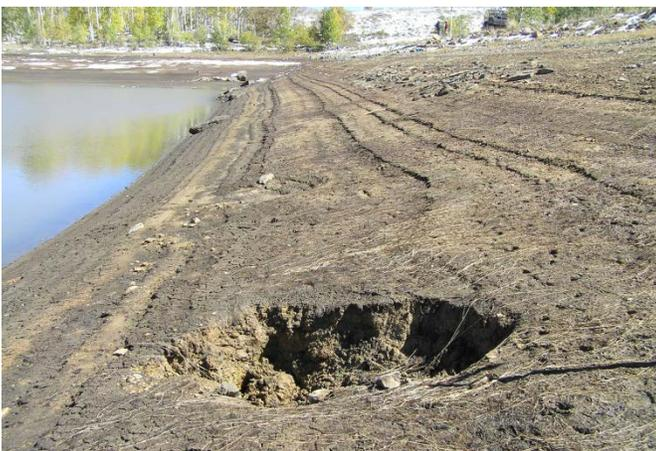
Photo 3: Sinkhole on upstream embankment (Paxton Dam)
