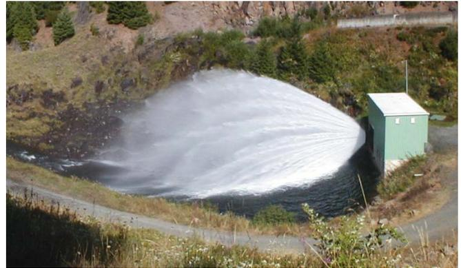
Photo 5: A cone valve dissipates energy downstream of an outlet works
