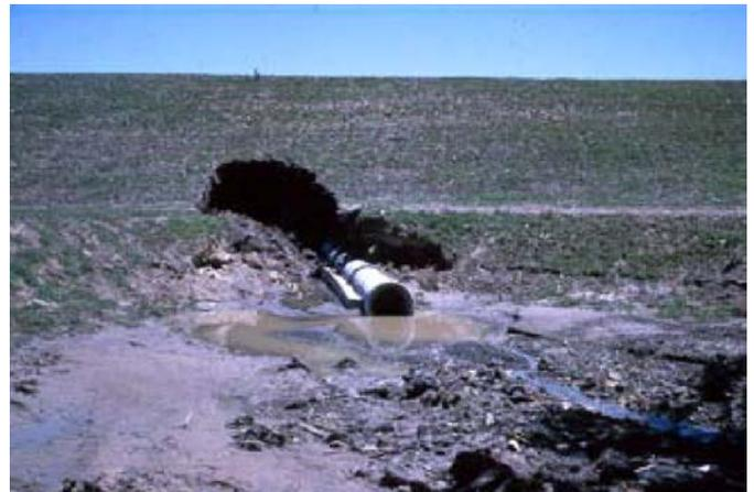
Photo 4: Piping failure along outlet conduit
