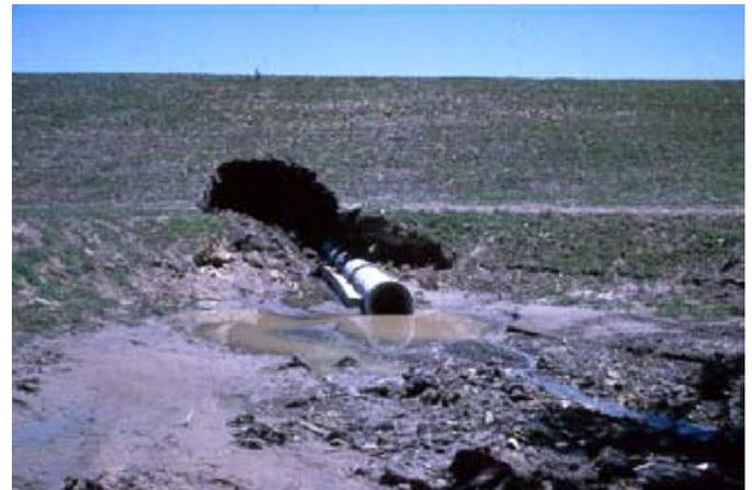
Photo 4: Piping failure along outlet conduit
