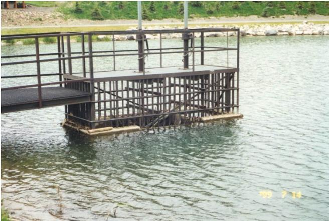
Photo 2: Trash racks surrounding an intake structure
