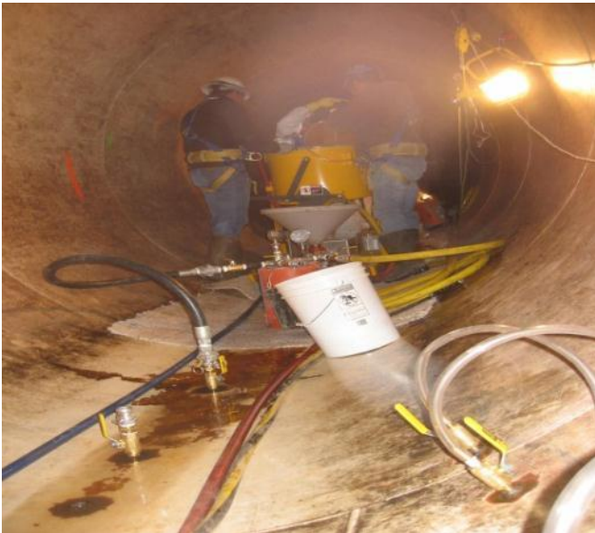
Photo 9: Injection grouting voided encasement behind steel liner.
