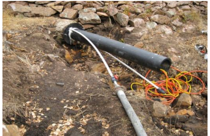
Photo 10: Grouting HDPE liner pipe. 3
