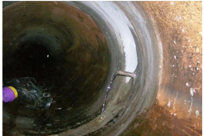
Photo 6: Grouted joint offset with grout port installed for injection grouting behind conduit.
