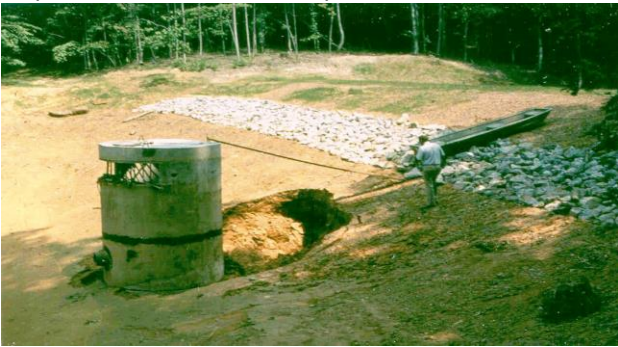
Photo 1: Sinkhole around a spillway riser 2
