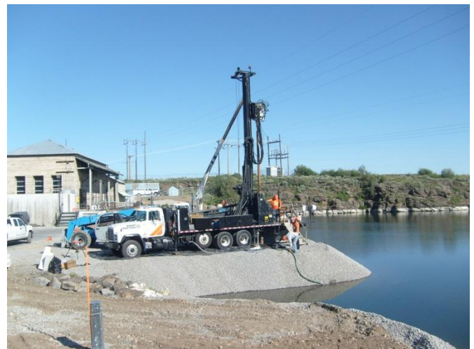
Photo 6. Sonic Drill Rig
