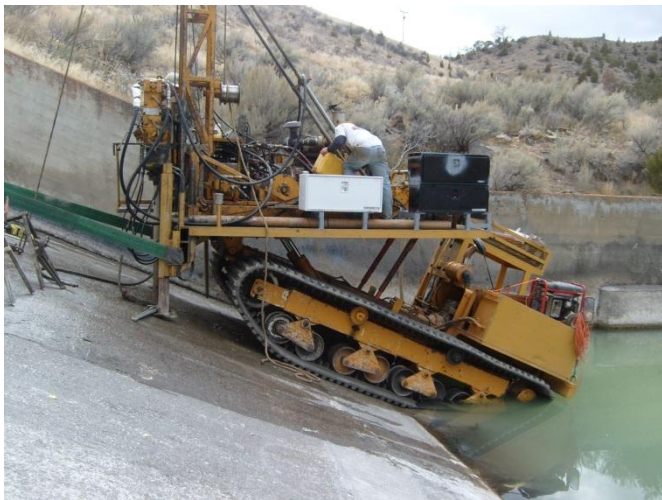
Photo 3. Core Drill Rig
