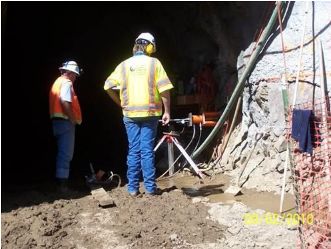
Photo 3. Contractor testing rock bolts with engineer oversight
