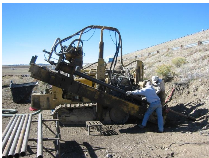
Photo 5. Odex Drill Rig
