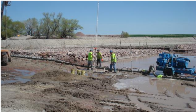
Photo 1. Site dewatering for a dam in South Dakota using well points.
