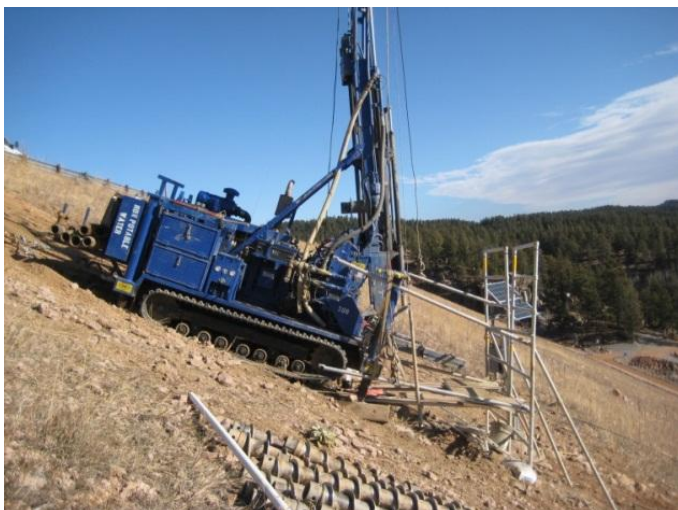
Photo 2. Auger Drill Rig
