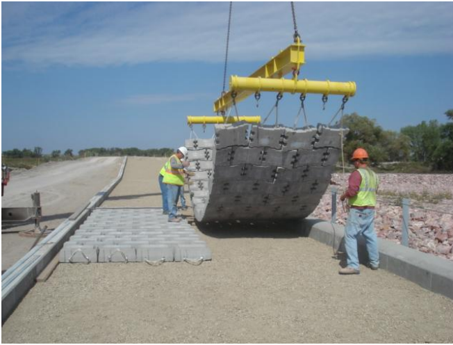
Photo 2. Prefabricated concrete armor mats for the crest of an overflow spillway.
