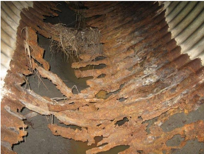
Photo 1: Severely deteriorated CMP. 1
