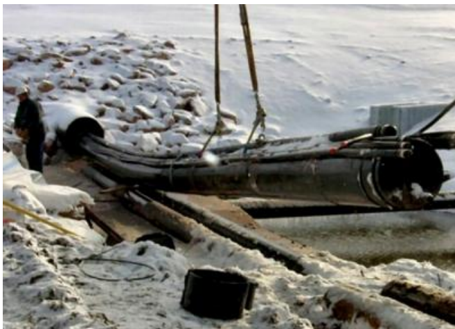
Photo 2: Installing HDPE Liner pipe. 2
