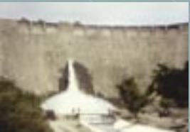
St. Francis Dam during failure, near Los Angeles, CA (1928)
