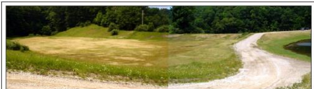
This open-channel emergency spillway is clear of trees, brush and other obstructions. Also note the good grass cover.
