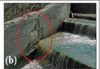
(a) The steel poles were used to hold a fish screen; the dam nearly failed during a flood because the screen collected debris and obstructed the spillway. The poles and screen were directed to be removed. (b) Spalled concrete can expose reinforcing steel, which can lead to rapid deterioration.
