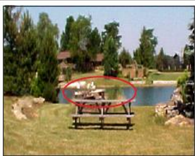
Notice the landscaping directly behind the table. Obstructions in the spillway reduce the capacity to convey water. They also can collect debris, further diminishing the capacity of the spillway.
