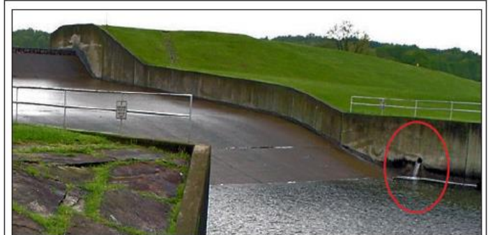
A properly designed spillway includes a drainage system for collecting seepage under the spillway. The picture shows flow discharging from the spillway's drainage system.
