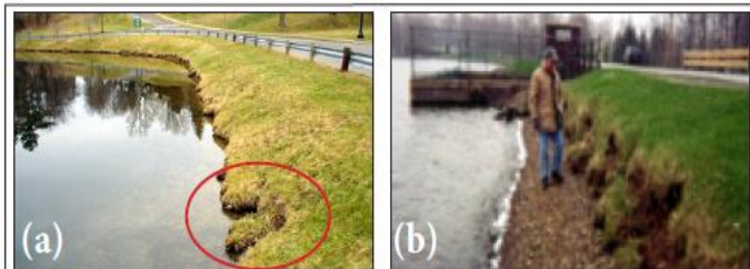
(a) Collapsed muskrat burrows increase shoreline erosion and sloughing. (b) This shoreline has eroded due to lack of proper erosion protection leading to sloughing and cracking of the slope.
