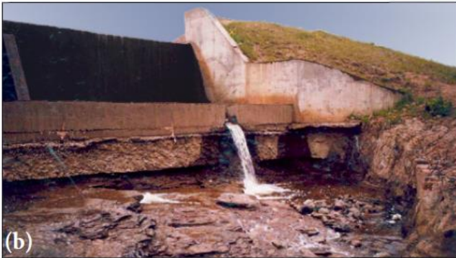
(a) A spillway outlet area as originally constructed. (b) Severe erosion has undermined the spillway outlet and threatens the overall structural safety of the spillway.
