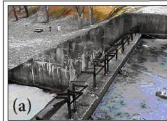
(a) The steel poles were used to hold a fish screen; the dam nearly failed during a flood because the screen collected debris and obstructed the spillway. The poles and screen were directed to be removed. (b) Spalled concrete can expose reinforcing steel, which can lead to rapid deterioration.
