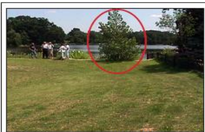
A tree is obstructing this spillway.
